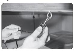
**Step 8:** Pull down on the ratchet rope, lifting the unit in place. We recommend pulling down on each individual ratchet rope 6-12 inches at a time until level.
