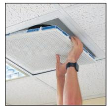
Lift face up and close. Secure by turning the two plastic screw heads with a coin or screw driver.
