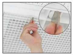
Use coin or screw driver to turn the two plastic screw heads and release the eggcrate return face
