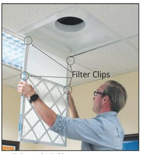
Slide 1" thick filter onto eggcrate face, sliding through filter clips...
