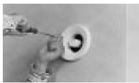
1.2 Using the appropriate hole cutting tool, cut a 4-1/8" diameter hole through the siding, sheathing, insulation and interior wall surface. Be careful to properly align the holes on the interior surface with the exterior, and ensure a slight slope towards the outside.
