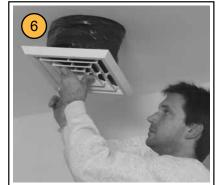
Push the diffuser and flexible duct into opening until grille contacts the ceiling. Rotate unit until it is parallel with walls in the room.
