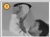
Choose an area free of obstructions (joists, electrical wires, etc.) for location of diffuser. For 6,7,8 inch boot mark a 9-1/4" diameter hole in the ceiling. For 4,5,6 inch boot mark a 7-1/8" hole. Cut hole using desired method (hand saw, utility knife,
