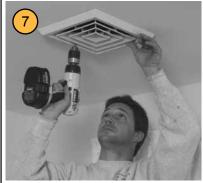
Tighten four screws until the unit is firmly secured in the ceiling. Clips will automatically swing to proper position.
