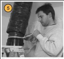
Slide duct over a collar and secure using tie wrap (provided). Tighten using tie wrap tool or pliers
