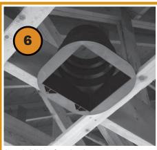
Attach MH to framing by screwing through provided openings below stand-offs.
