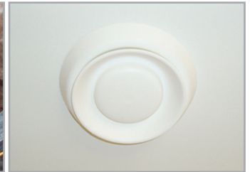
Finished installation with Primex WG Series Diffuser
