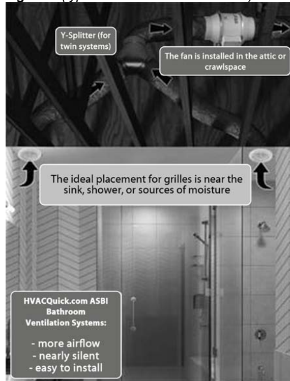
Figure 1 (typical bathroom kit installation)
