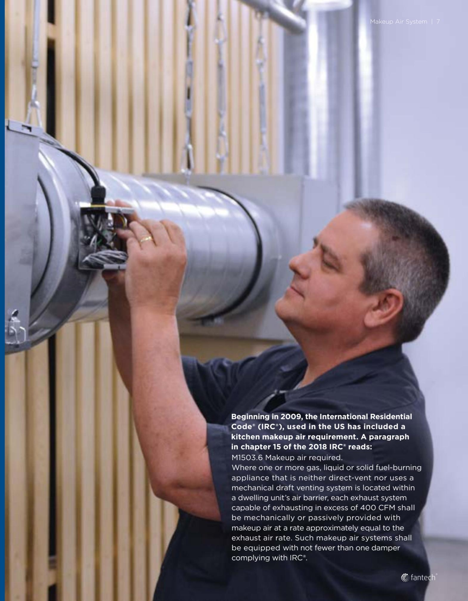
**Beginning in 2009, the International Residential Code® (IRC®), used in the US has included a kitchen makeup air requirement. A paragraph in chapter 15 of the 2018 IRC® reads:**
